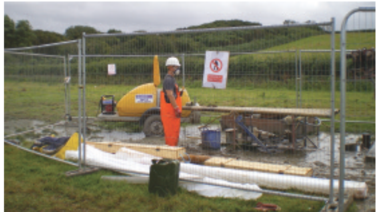
Drilling boreholes at Hinkley Point
